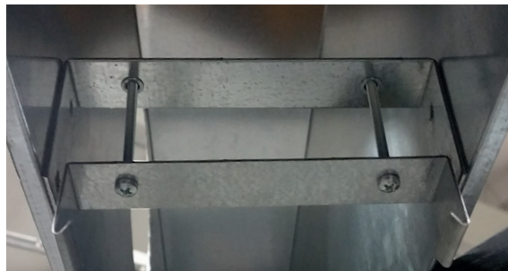
Sliding U-BRACKETS in optimal position during the LINEAR DIFFUSER installation.
